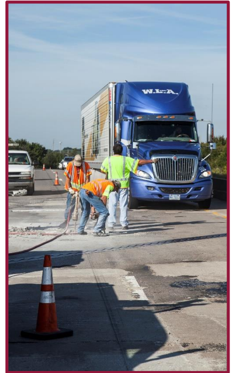
Figure 10: Maintenance on Oklahoma Roadway
