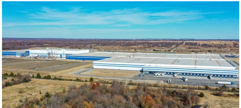
Figure 2: Sofidel's Inola facility under construction.
